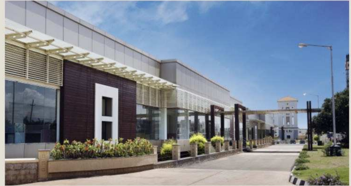
Sobha Manufacturing Unit
